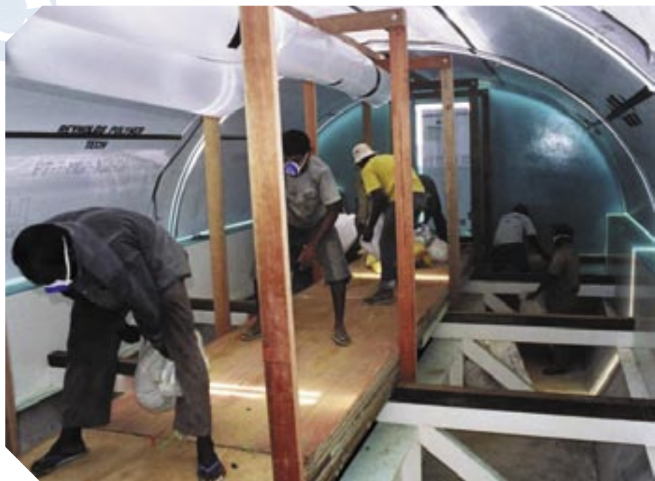
Local workers manhandle sandbags into position for sinking.
