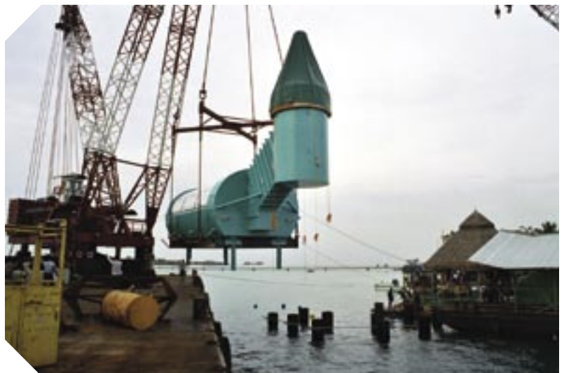
A barge with a 300-tonne crane transported the structure from Singapore.
